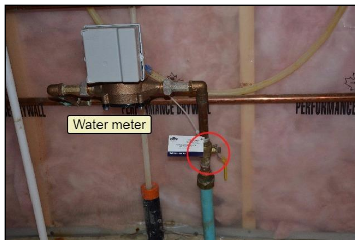
77. Main water shut-off valve
