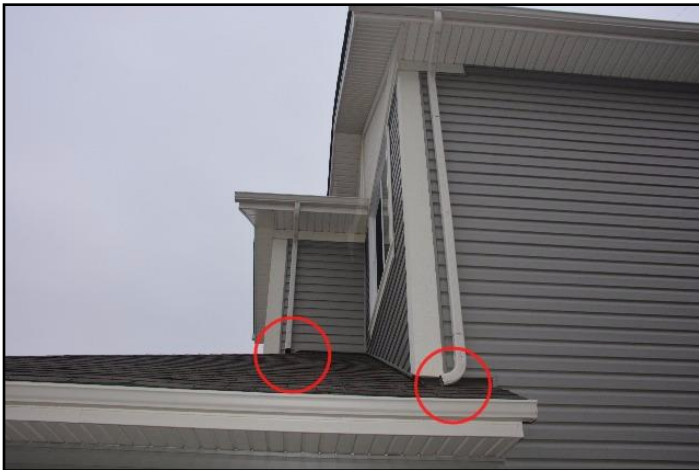
18. Downspouts discharging onto roofs
