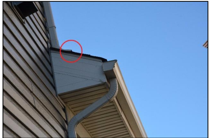
19. Downspouts discharging onto roofs
