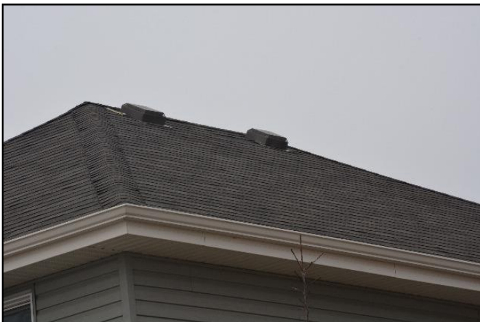
1. Asphalt Shingles. Top roof
