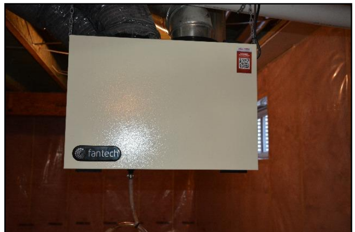
63. Heat recovery ventilator (HRV)
