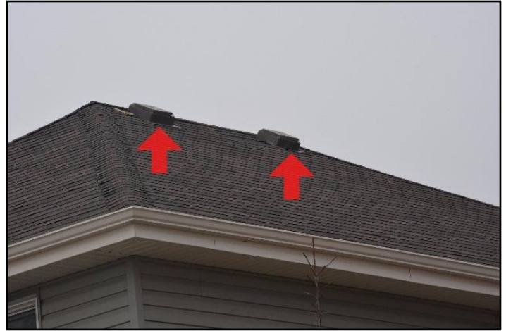
15. Loose flashing
