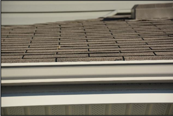
5. Asphalt shingles. Garage roof
