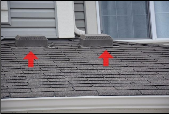
14. Loose flashing
