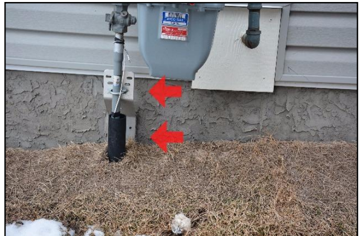
36. Typical minor cracks
