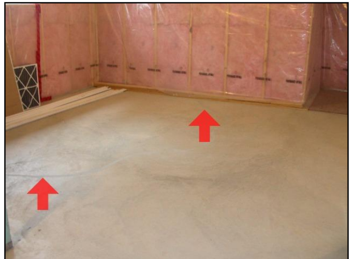
40. Crack (repaired)
