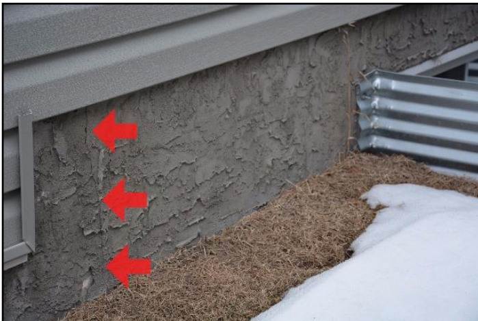
35. Typical minor cracks
