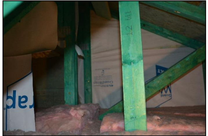
68. Garage roof insulation
