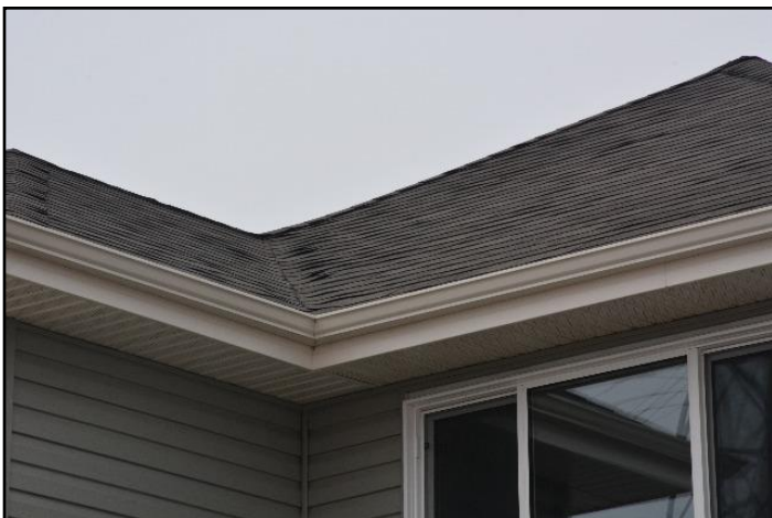
3. Asphalt Shingles. Top roof
