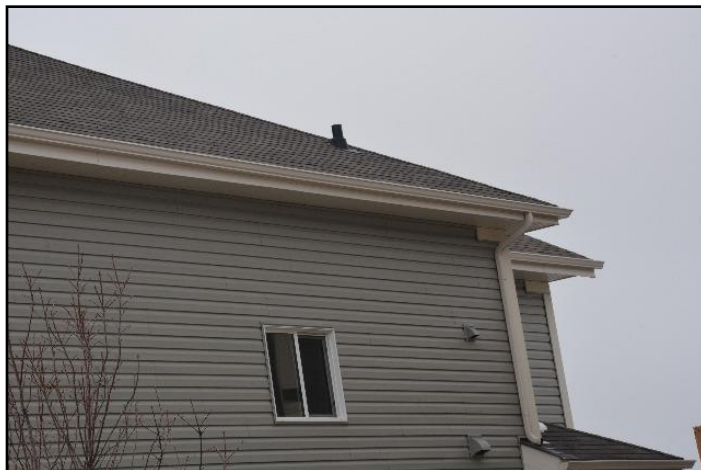
2. Asphalt Shingles. Top roof
