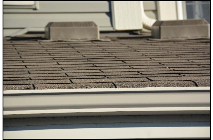
6. Asphalt shingles. Garage roof
