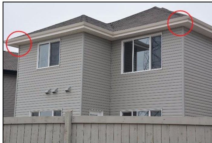
20. Downspout missing
