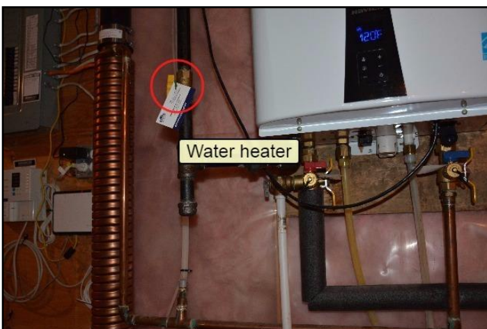
53. Gas shut-off valve
