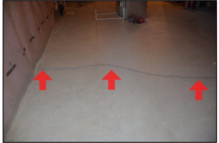
38. Crack (repaired)
