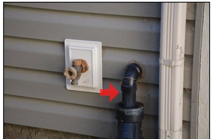
81. Sump pump discharge
