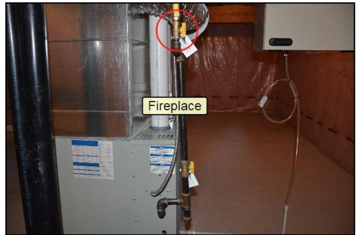
56. Gas shut-off valve
